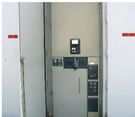
Before: full voltage starter
