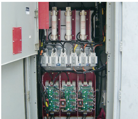
After: Solid state reduced voltage starter
