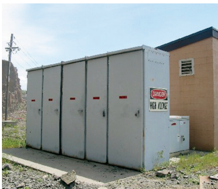
5 kV medium voltage lineup
