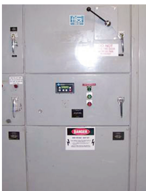
After: solid state reduced voltage starter
