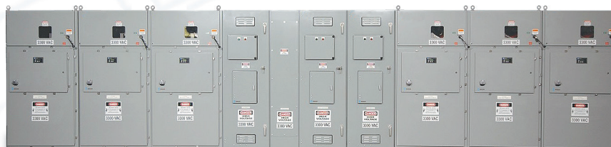
Draw Out Circuit Breaker MTM with (6) 5 kV solid state starters
